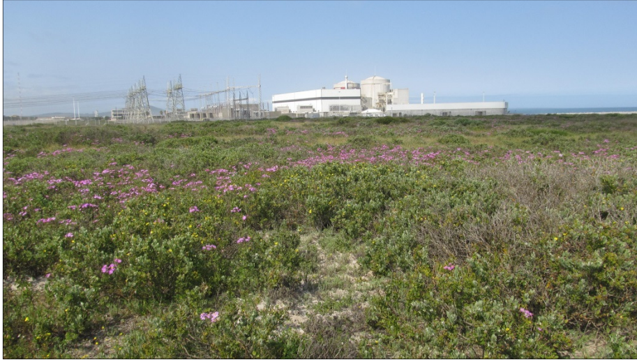
Figure 4. View of the proposed development site.
